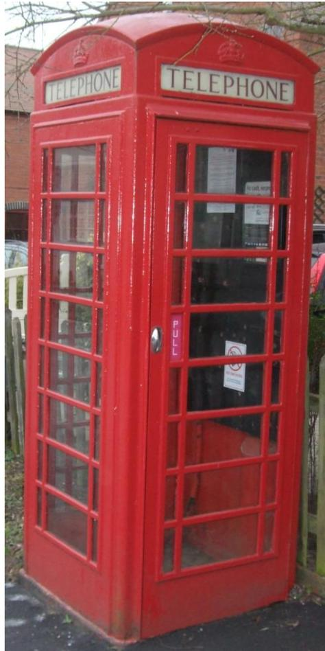
The door was repositioned when the telephone box was moved from outside the Post Office. The door is actually made of teak – the metal glazing bars & slow closing mechanism help to give the impression of weight.
